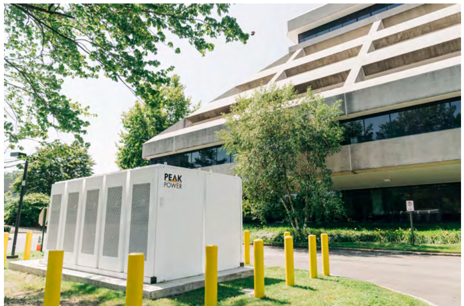
Battery storage project in Westchester, NY
